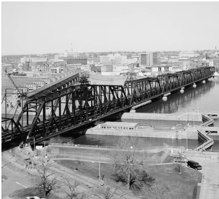
Rock Island Arsenal (or Government) Bridge, 1985 Connecting Rock Island, IL to Davenport, IA by rail (and road on lower level) at Lock and Dam No. 15
