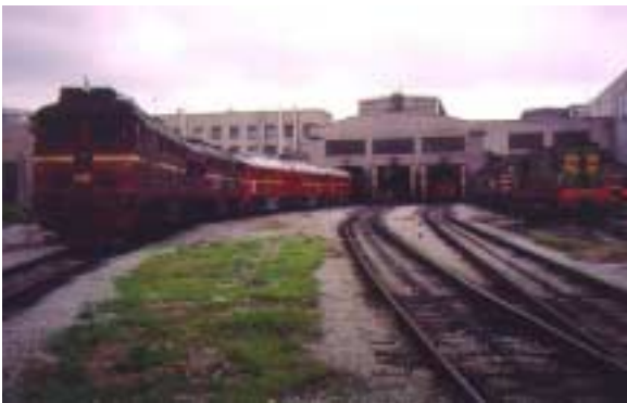
EVR's principal locomotive maintenance works is located at the key junction of Tapa
