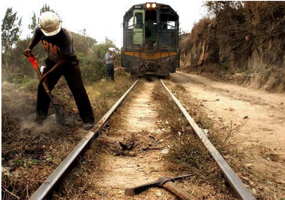
A worker puts out a fire on the tracks en route to the coast. Bandits set fire to the railroad ties to loosen the metal of the tracks, which they sell for scrap. (Sarah Meghan Lee / For The Times)
