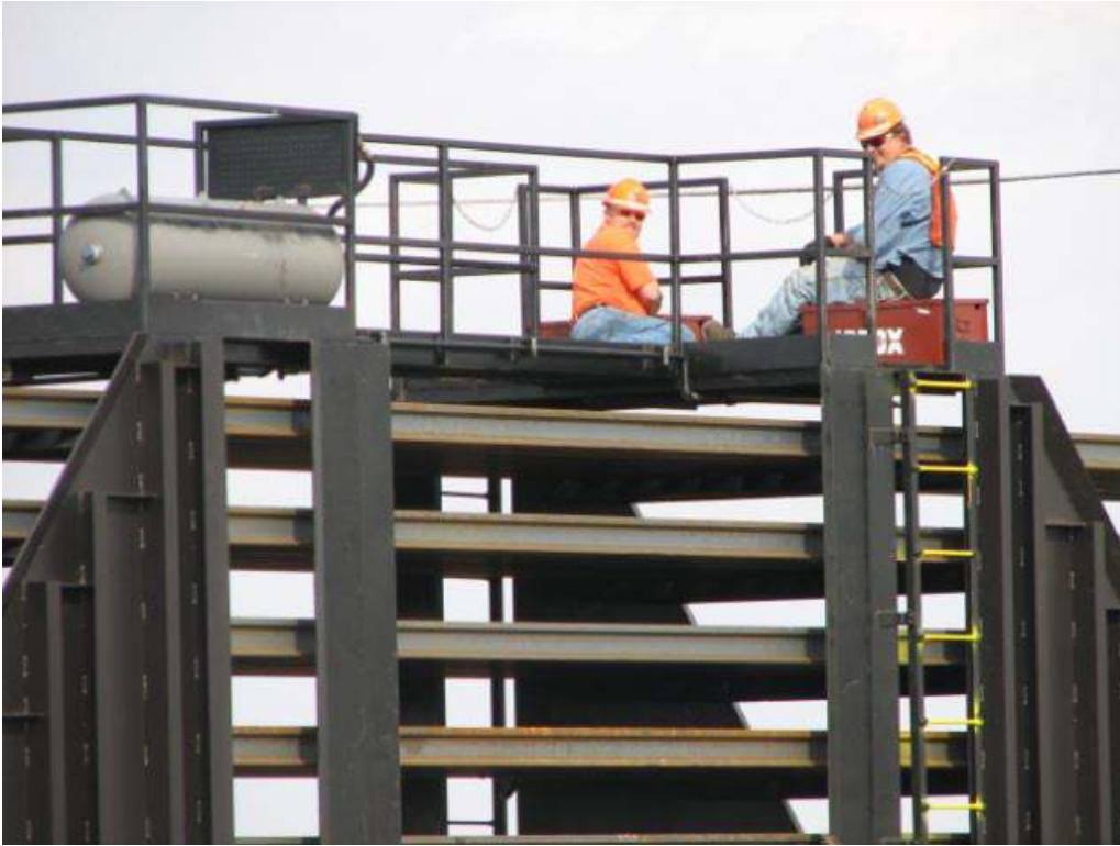
Above: IAIS crews deliver and unload the rail ribbon in Annawan.
