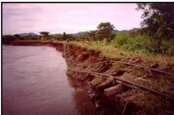
After Hurricane Mitch, additional storms hit us and this is what our mainline looked like after it had been rehabilitated. Needless to say, we had to go back and do this work all over again, at least in terms of replacing the embankment.
